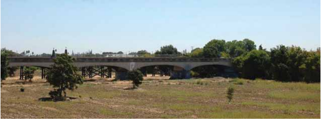
Figure 2.1.4-2 KV 1 – Existing Condition
