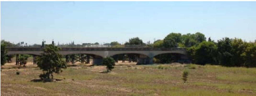
Figure 4 Existing Conditions at TRRP Gateway Parcel
