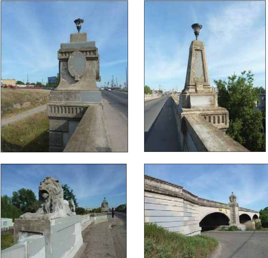
Figure 2.1.5-1 Representative Architectural Features
