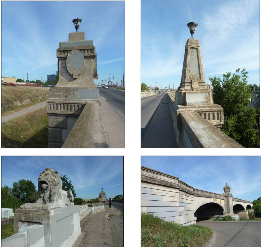
Figure 2.1.5-1 Representative Architectural Features
