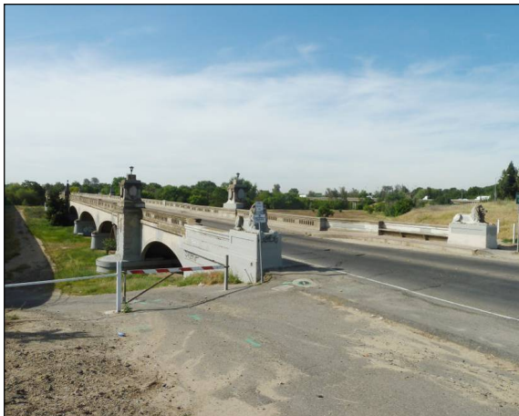
Figure 2 7th Street Bridge from the North Bank of the Tuolumne River (facing southwest)
