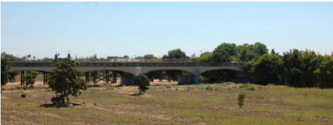
Figure 4 Existing Conditions at TRRP Gateway Parcel
