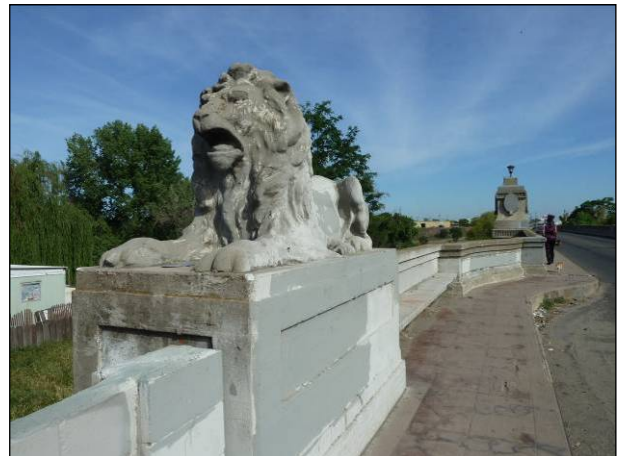
Figure 3 Recumbent Lion at the Southwest Corner of the Bridge with Concrete Bench Behind It (facing northwest)
