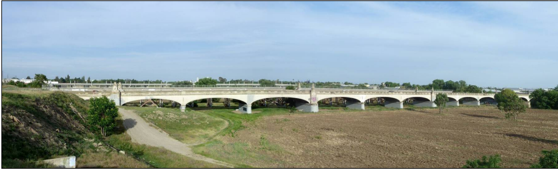
Figure 1 7th Street Bridge from the North Bank of the Tuolumne River (facing southeast)
