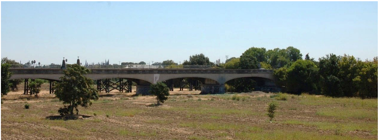
Figure 2.1.4-2 KV 1 – Existing Condition
