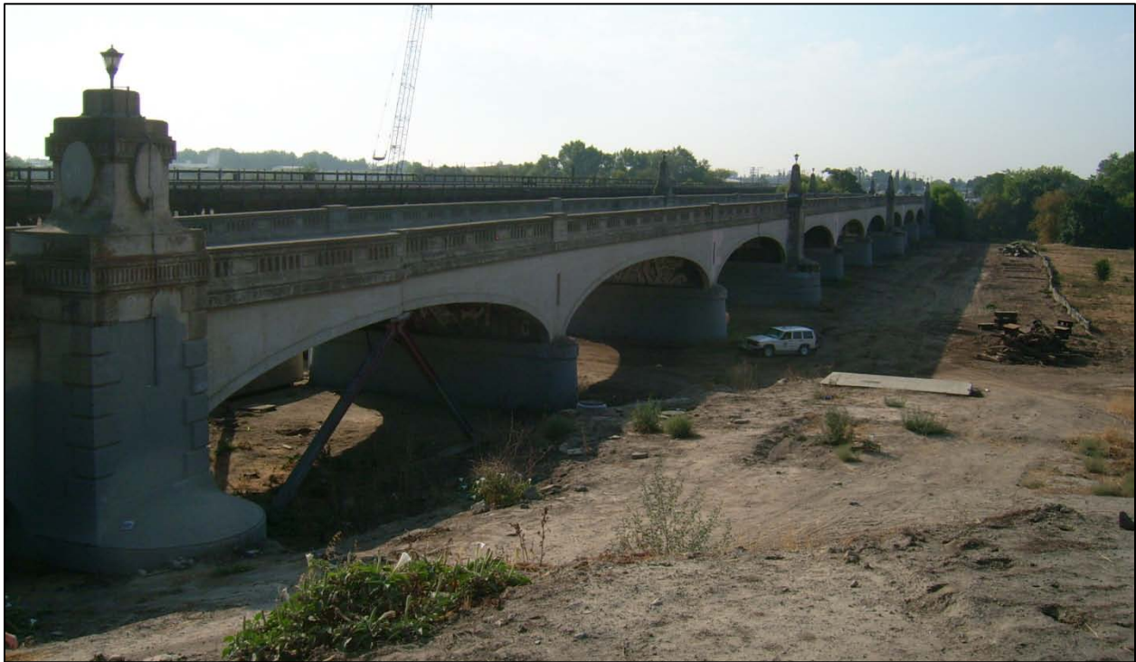
Figure 3 – West Edge of Bridge Looking South
