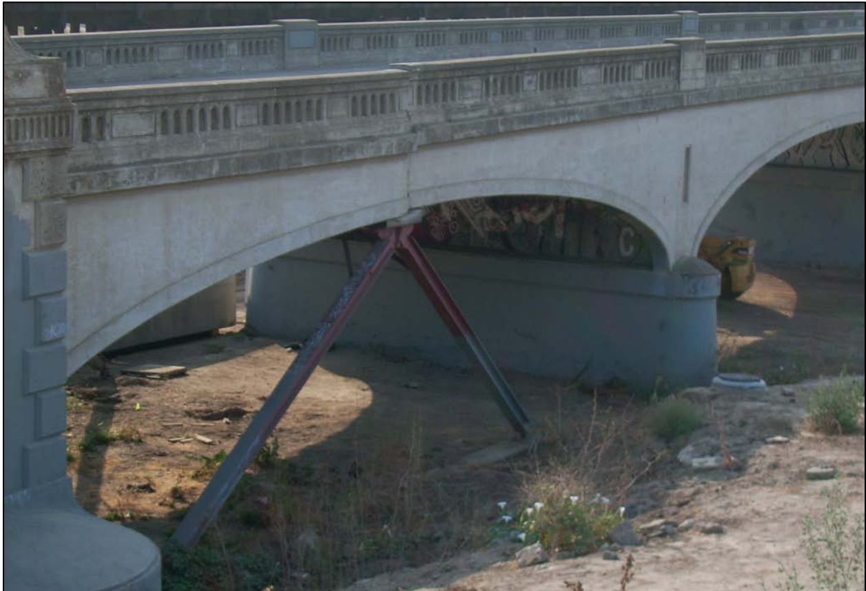
Figure 4 - Span 13 Support at Joint
